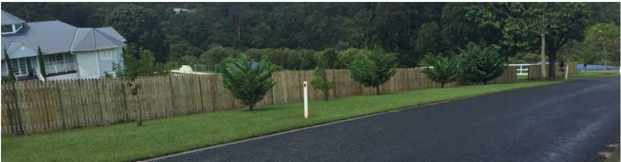
Timber picket fence
